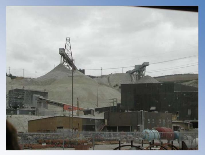
1. The mill complex is a major structure at an operating mine (dark grey building, centre right). Here coarse ore conveyed from the primary crusher and stockpiled nearby, is broken up further to fine particles and separated from waste rock sand. In the case of sulphide ore deposits, like those of copper, molybdenum, and lead, sulphide - *concentrate* is separated from the *tailings* in the mill.
