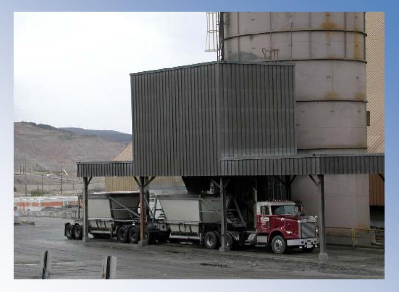
13. Dry concentrate is stockpiled in a shed before being shipped to market, here via covered truck, then to a railway.
